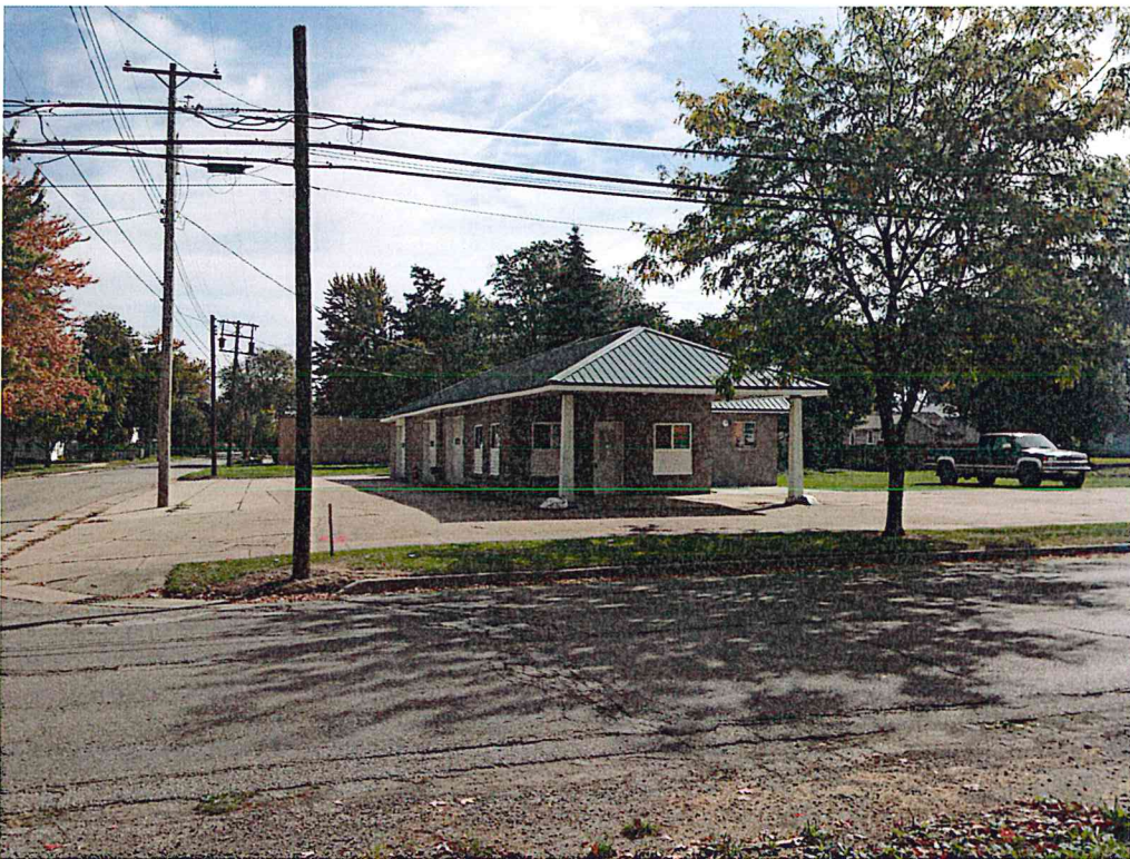
NORTHWEST PROPERTY CORNER – FACING EAST OFF LANSING STREET
