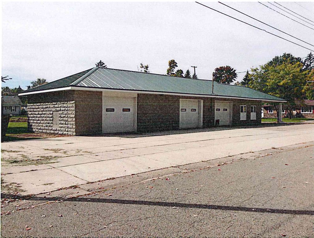
NORTH PROPERTY LINE – FACING SOUTHWEST OFF STEEL STREET
