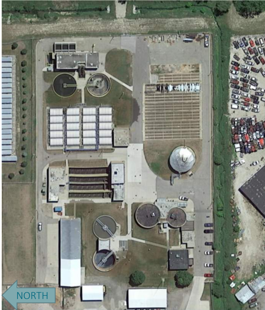
Aerial View of Existing WWTP
