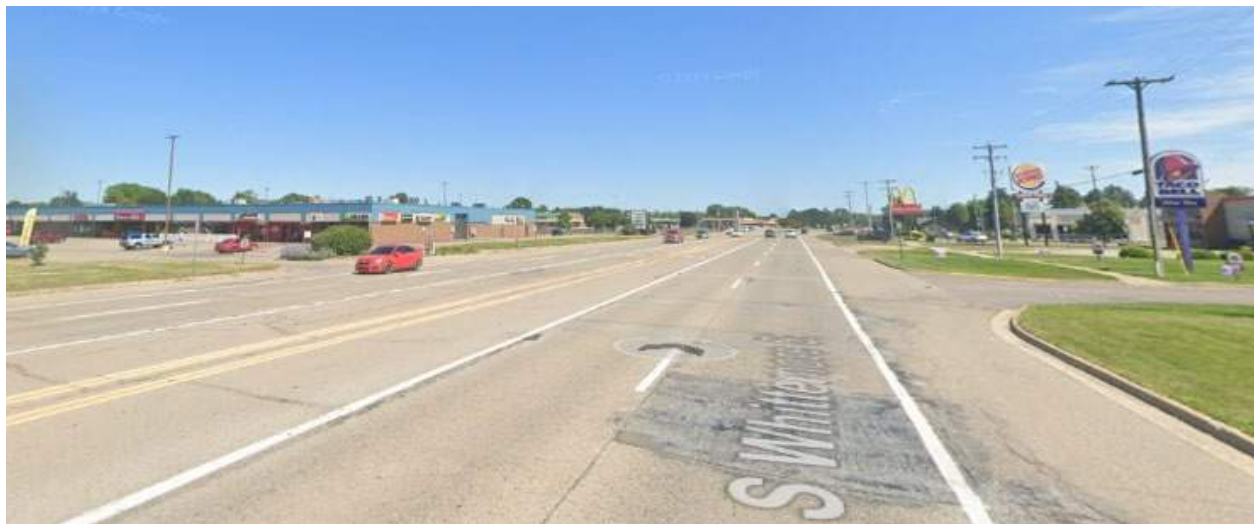
The US 127 right-of-way is 180' across, with 4 travel lanes, 2 center turn lanes, and 2 large shoulders.
