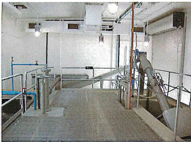
Aerated Grit Tank and Screening Equipment
