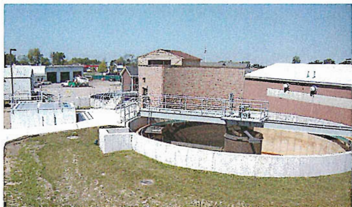
One of two new 45-foot diameter clarifiers.
