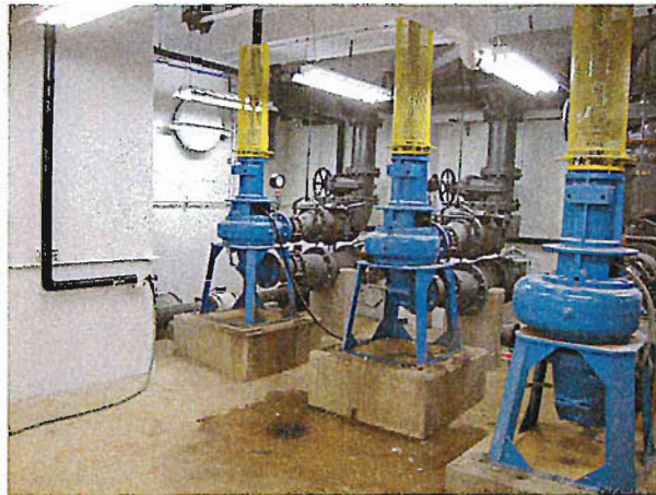
Improvements to raw sewage pumping provide firm capacity of 10.5 MGD to accommodate the peak hour flows
