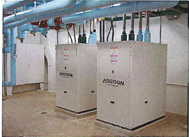
Water-to-water heat pumps in the Grit/Raw Sewage Pumping Building
