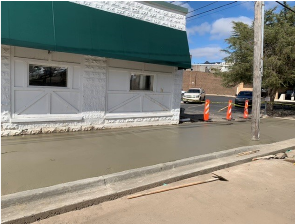
Concrete and curb & gutter – Higham & Brush Streets
